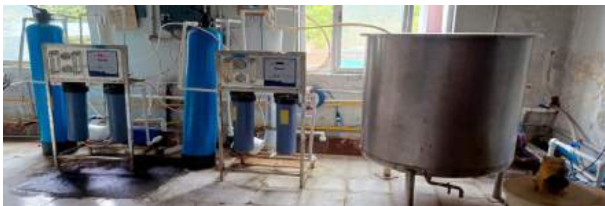
Fig : Installation of RO Plant in Main Building of BCGVL
