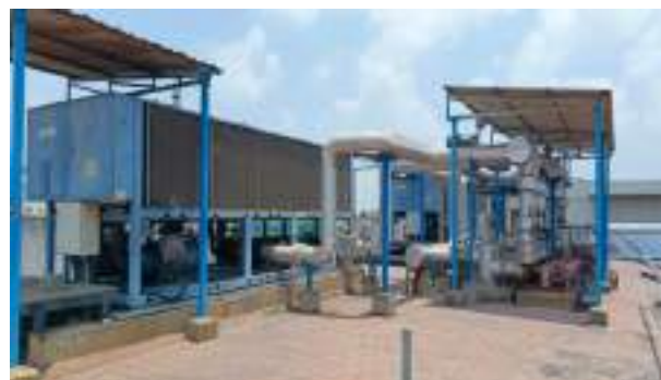
Fig : Air Cooled Chiller
