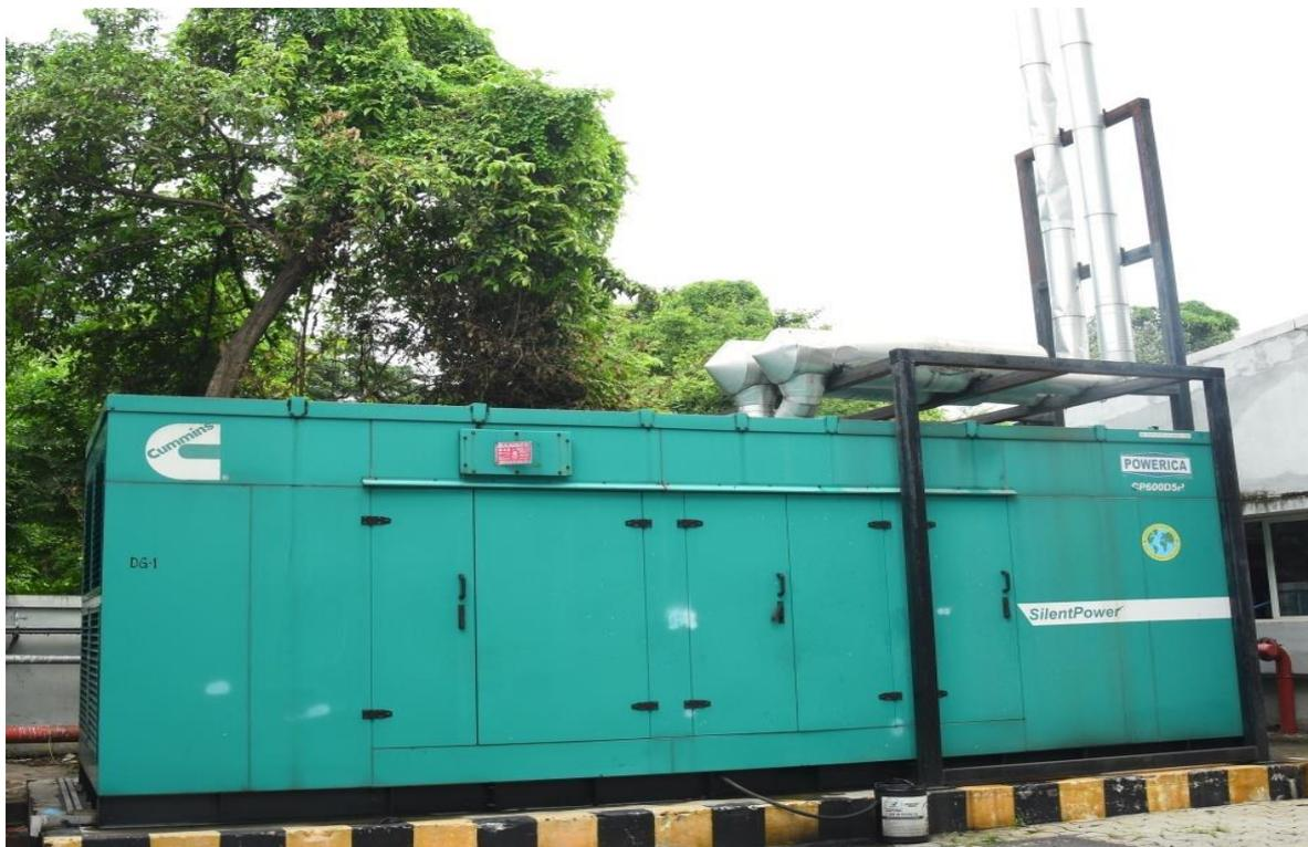
**Diesel Generator with 600KVA capacity**
