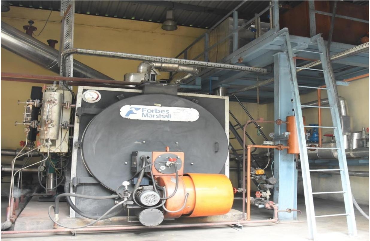
**IBR Boiler with capacity 1.5 tonne**
