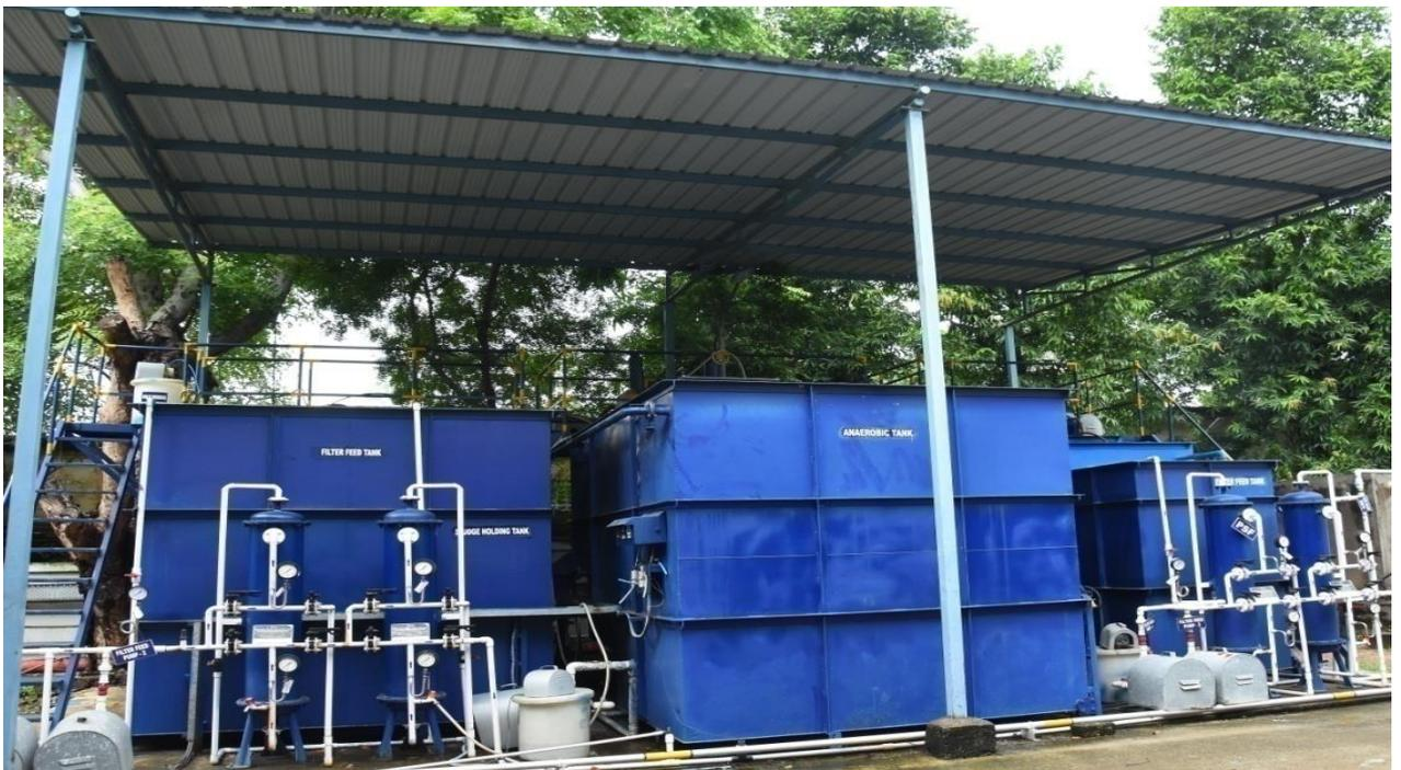
**Effluent Treatment Plant (15KLD capacity) and Sewage Treatment Plant (4KLD capacity)**
