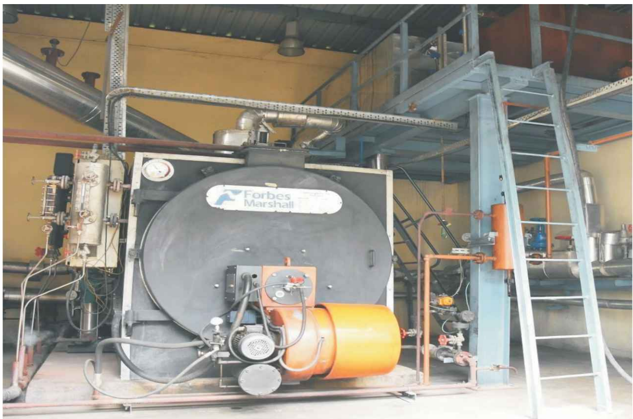
IBR Boiler with capacity 1.5 tonne
