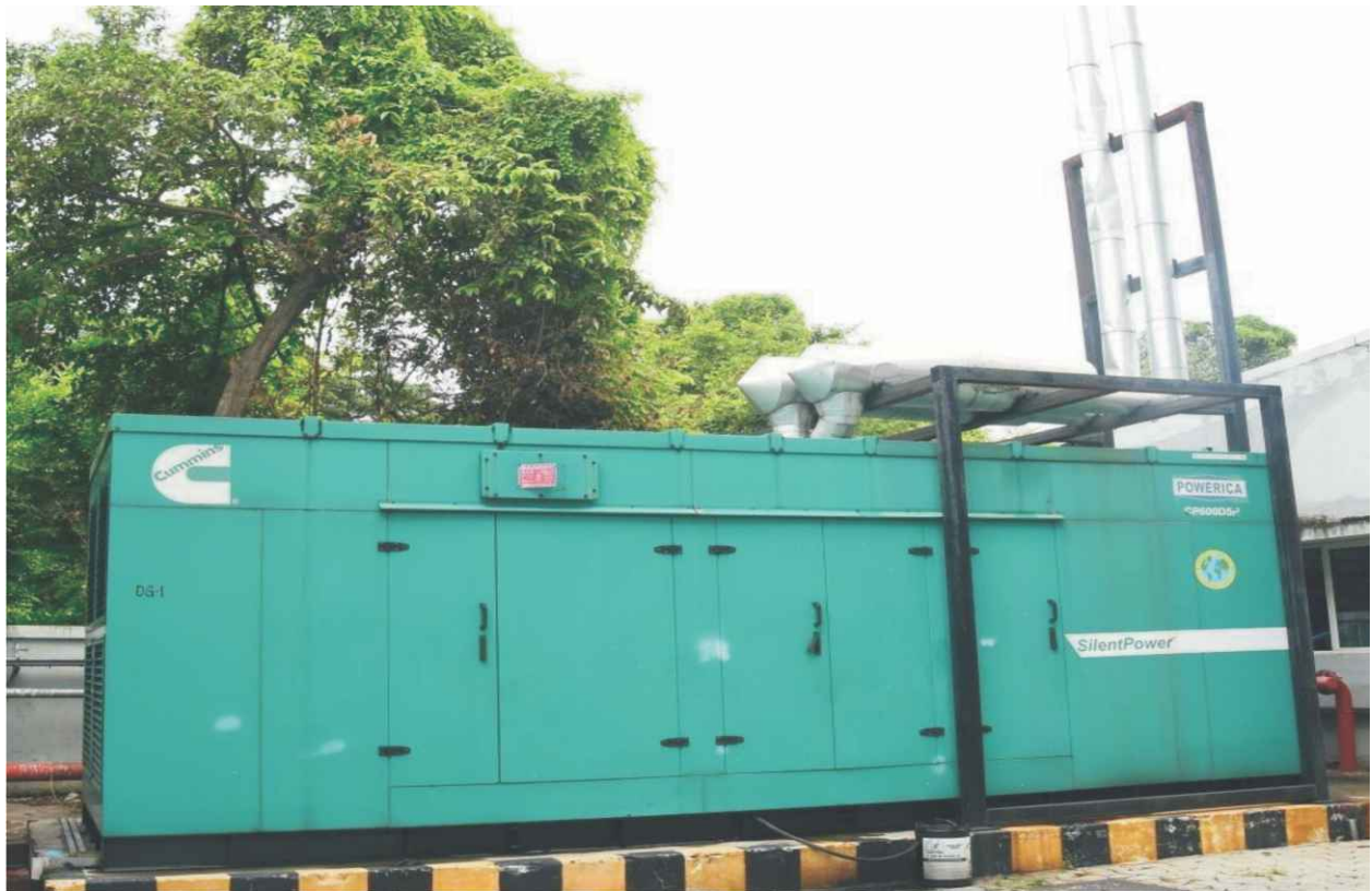
Diesel Generator with 600KVA capacity
